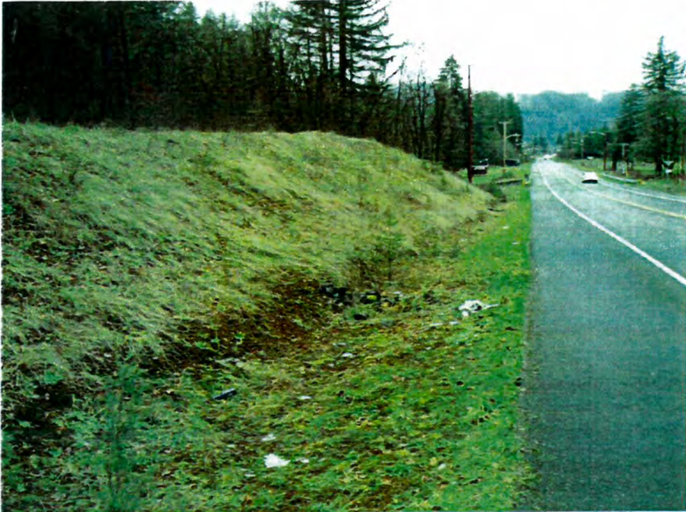
Slope along the southern end of the project.
