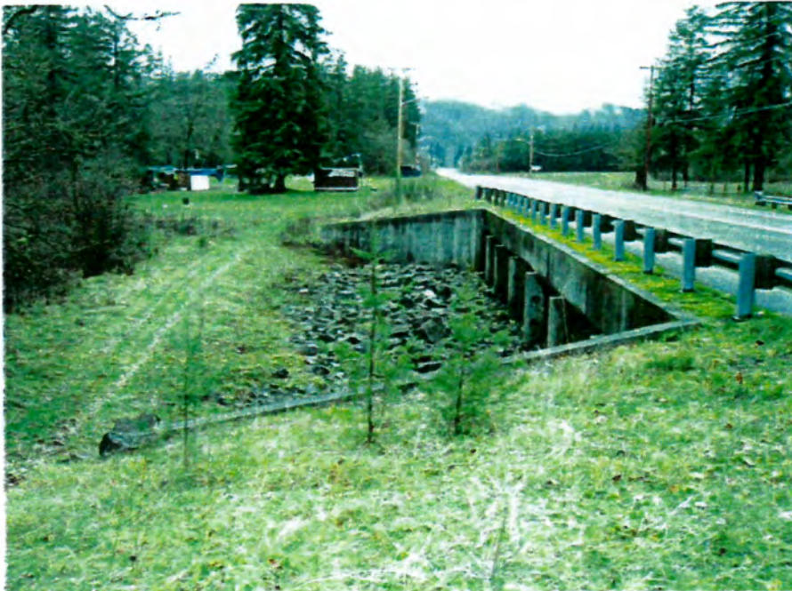
The southernmost set of Anderson Road culverts.
