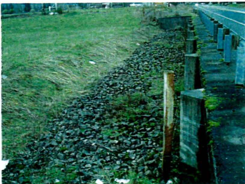
Culverts where floodwaters flow under Anderson Road.
