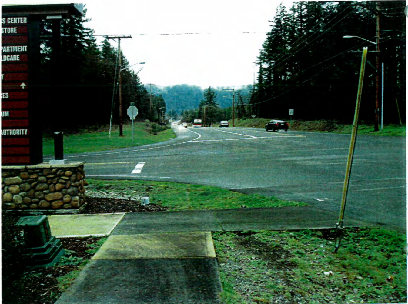
Looking north along Anderson Road, from the Howanut Road intersection.
