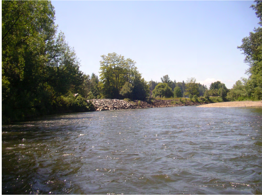
June 2008. Riprap placed on bank of Chehalis River by Thurston County, downstream of Independence Road bridge. Source: Herrera Environmental Consultants
