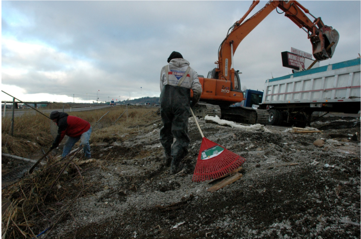
(FEMA, Debris after Washington Flood)
