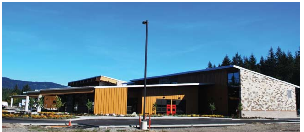
Tribal employees started moving into the new Chehalis Tribal Community Center on October 16. Although it is never fun to move, employees are excited about the quality and atmosphere of the building and offices.
