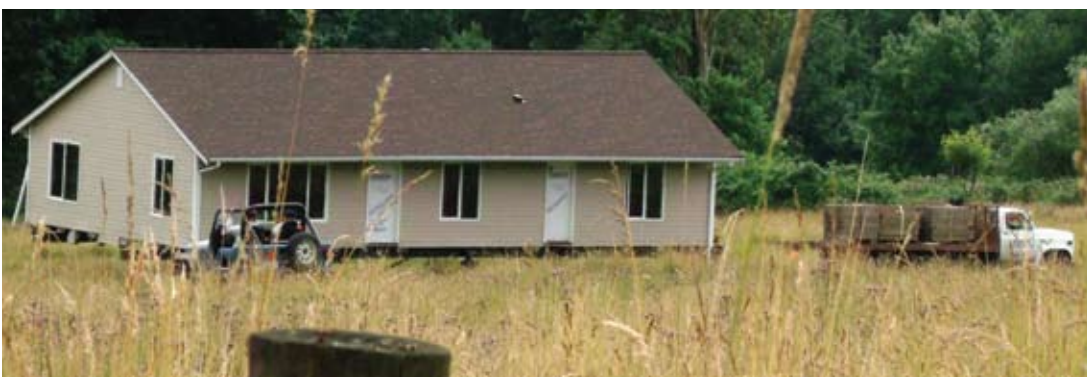
The Hard Rock Excavating Company moves a mobile home across the field to its final location across from the Fish Hatchery on Howanut Road. A new foundation is being built and will be available to rent to tribal members.
