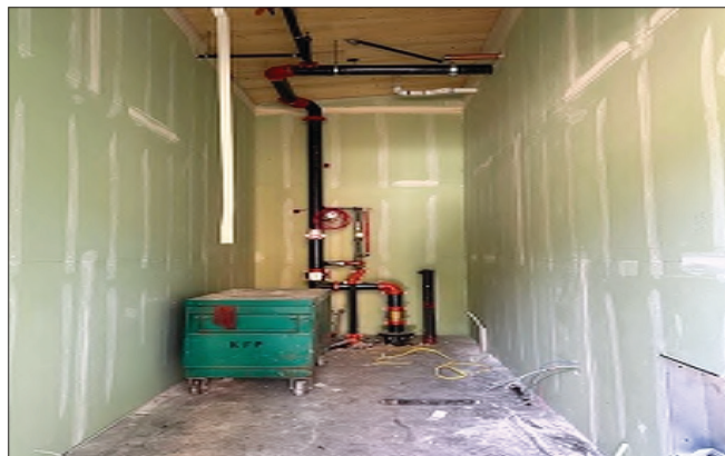
Above: Waiting room painting is completed. Left: The sprinkler riser room is taped.
