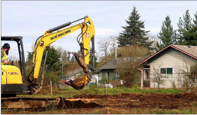
Work begins on the Chehalis Tribe's modular homes development in Oakville.
