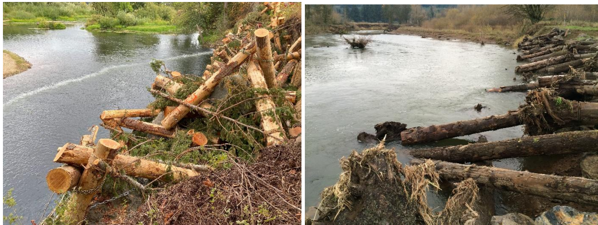
Figure 4.3 Engineered Large woody debris (LWD) used to stabilize bank erosion; on Newaukum River (left) and Chehalis River at Ceres Hill Rd. (right) (NHC, 2015, 2021).
