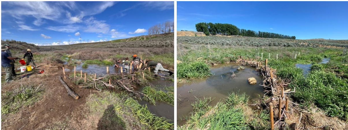
Figure 4.6 Photos of constructed Beaver Dam Analogs (BDAs) using post-assisted methods, during construction (left) and post-construction (right) (NHC, 2025).
