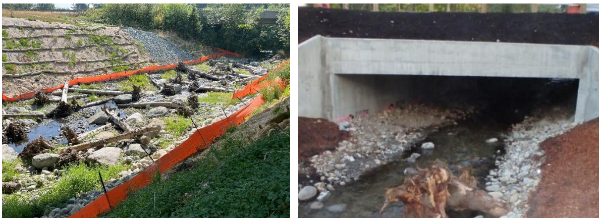
Figure 4.9 Post-construction examples of fish passage barrier replacement and riparian restoration projects in Western Washington (NHC, 2026a; WSDOT, 2015).
