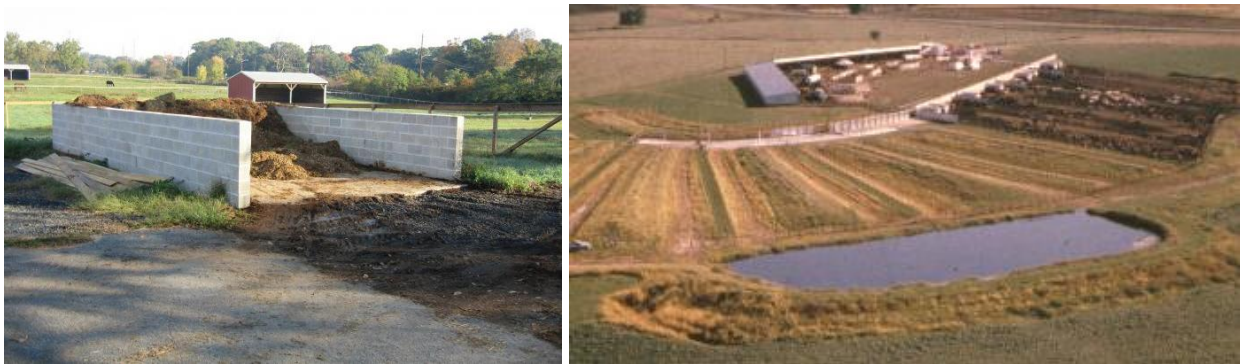
Figure 4.4 Photos of a livestock manure dry stack (left) and runoff holding ponds (right) used to improve the water-quality of runoff from agricultural operations (Livestock and Poultry Environmental Learning Community, 2019b, 2019a).
