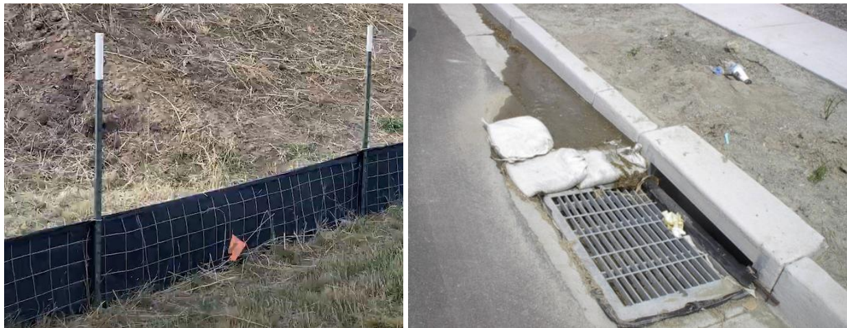
Figure 4.8 Construction site erosion and sediment control measures, silt fencing (left) and curb inlet protection (right) (Washington Stormwater Center and Minnesota Pollution Control Agency, 2026).
